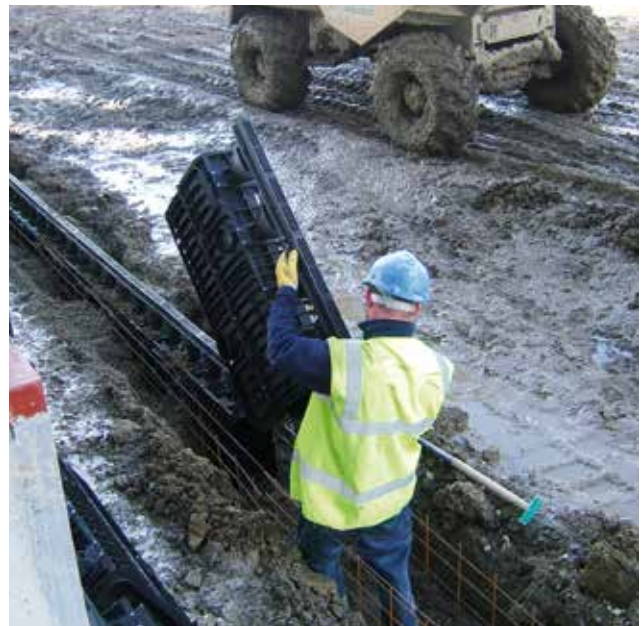
Lightweight elements, installed by one single worker.
