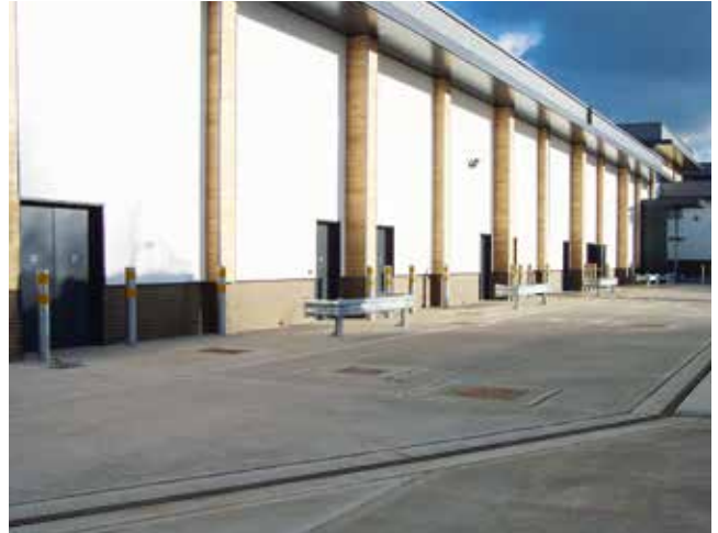
Installation in concrete surface
